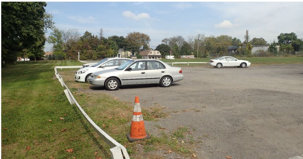
Gables Site Deficiency: Lack of ADA parking, curbing, directional arrows, parking delineation and asphalt paving
